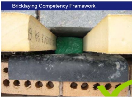
Installing Fire Breaks and Barriers
